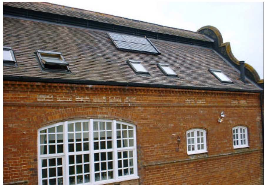
Examples of 1.86m 2 (2m 2 nom. aperture area) LaZer2 Domestic Solar Water Heating Systems
