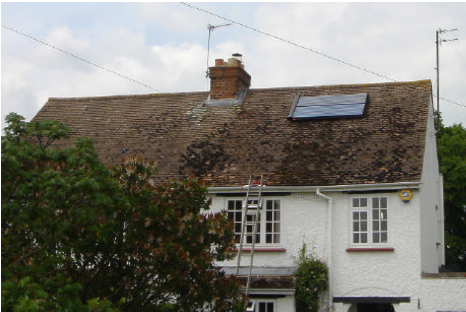
Examples of 1.86m 2 (2m 2 nom. aperture area) LaZer2 Domestic Solar Water Heating Systems
